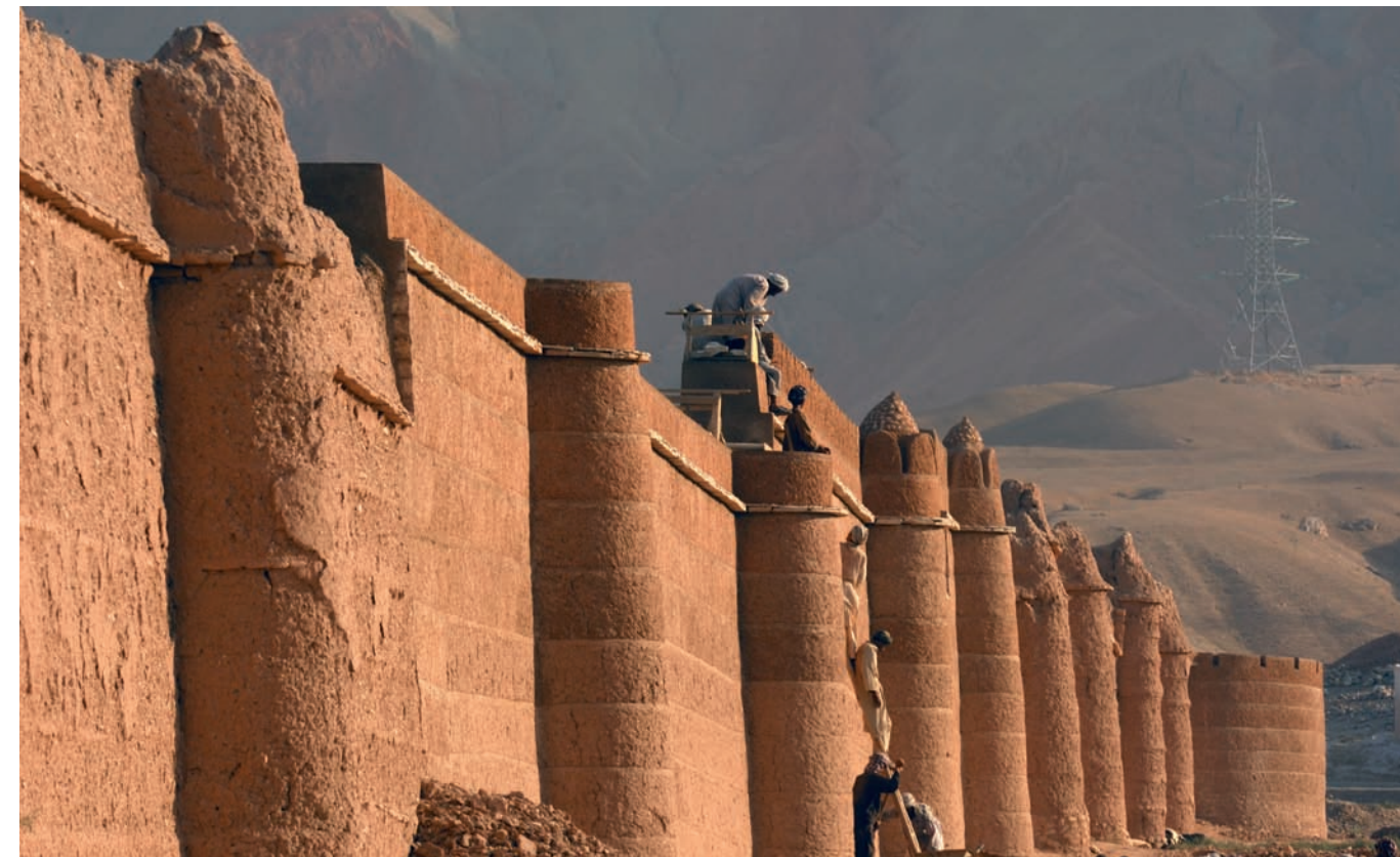
Building activities with the traditional pakhsa system at the palace garden wall of the Bagh-e Jehan Nama Palace.
