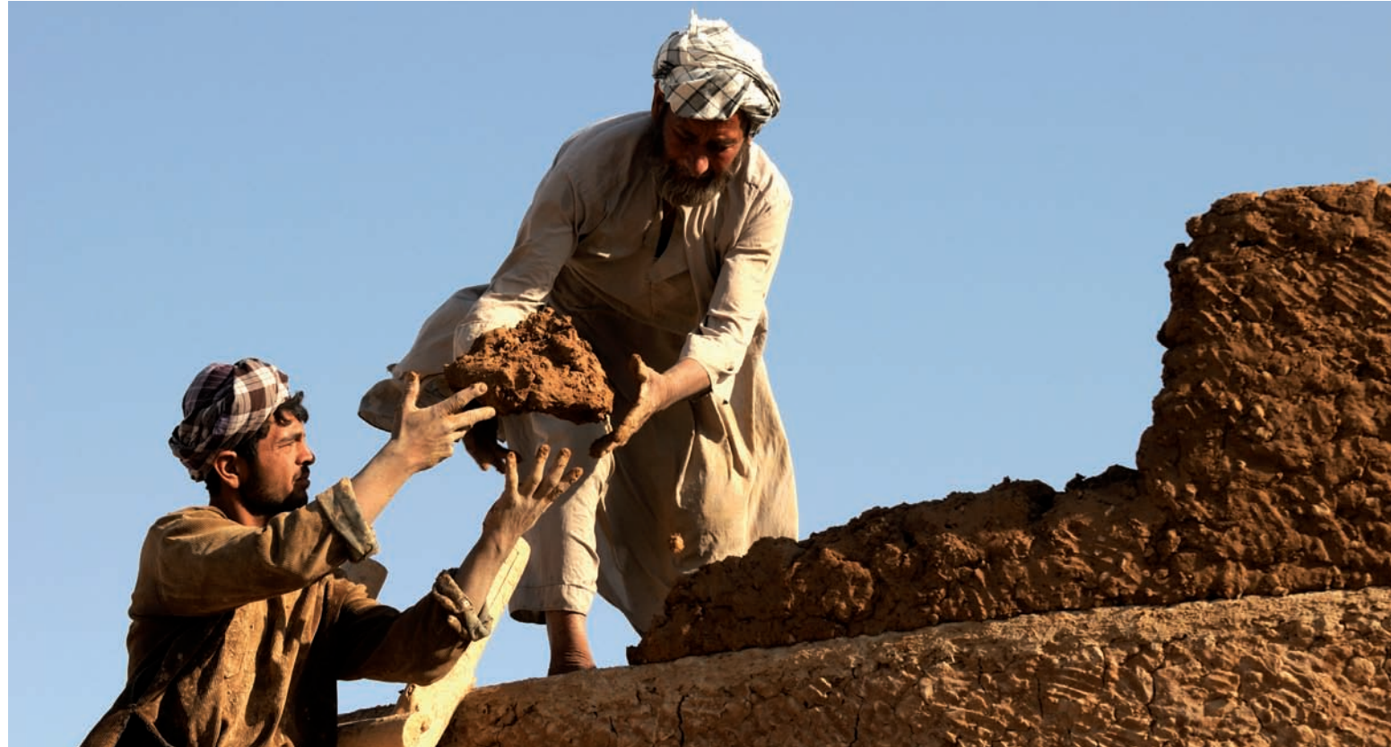
Making a new pakhsa layer on the garden wall of the Bagh-e Jehan Nama Palace.
