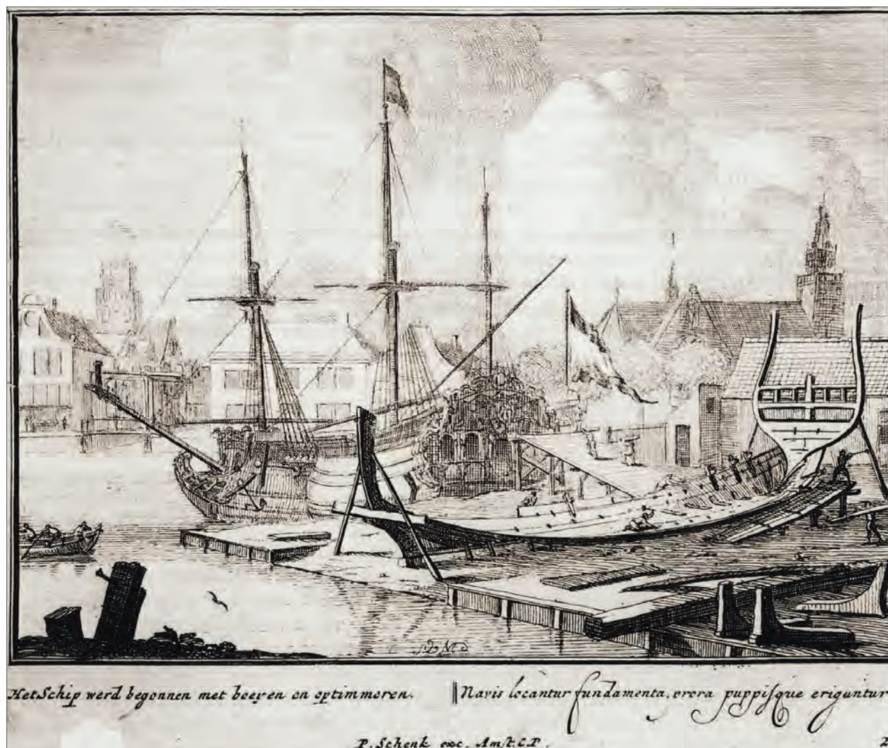
Figure 9.14 Drawing by Sieuwert van der Meulen from his series Navigiorum aedificatio from around 1700, showing the Dutch flush-planked shipbuilding (Groot & Vorstman 1980).
